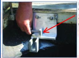
Install (2) 3/8" x 1 <sup>1</sup>/2" pivot bolts from the outside to inside of both pivot clevises until the end of the bolt is flush with the inside of each clevis. (Do not install the bolts past the inside edge of the clevis). The Retro-Grate<sup>TM</sup> will be positioned between the two pivot clevises and clearance for the grating structure must be maintained.
