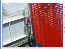
Grasp the spring loaded lifting handle and pull the Retro-Grate™ into the open and upright position. If the unit is installed properly, the red latch should move into a locked position beneath the slide angle and the grating structure cannot be lowered. If the latch does not move into the locked position, consult the factory. To lower the Retro-Grate™, grasp the lifting handle with one hand and with the other hand, simply pivot the red latch upward and lower the unit.
