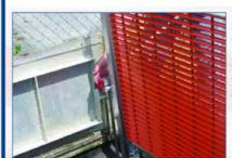
Grasp the spring loaded lifting handle and pull the Retro-Grate™ into the open and upright position. If the unit is installed properly, the red latch should move into a locked position beneath the slide angle and the grating structure cannot be lowered. If the latch does not move into the locked position, consult the factory. To lower the Retro-Grate™, grasp the lifting handle with one hand and with the other hand, simply pivot the red latch upward and lower the unit.
