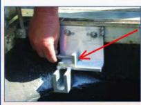
Install (2) 3/8" x 1 <sup>1</sup>/2" pivot bolts from the outside to inside of both pivot clevises until the end of the bolt is flush with the inside of each clevis. (Do not install the bolts past the inside edge of the clevis). The Retro-Grate™ will be positioned between the two pivot clevises and clearance for the grating structure must be maintained.
